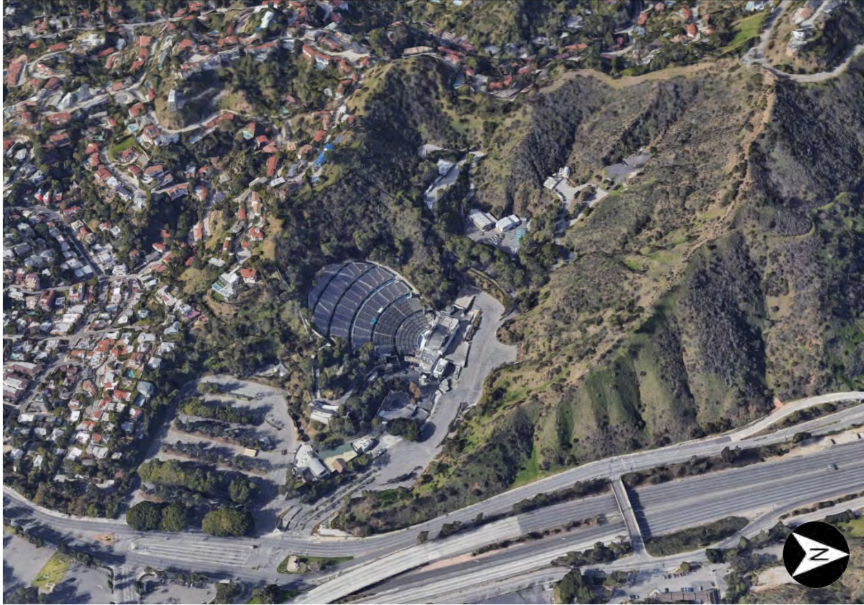
Figure 1 Aerial view of Bolton Canyon with the Hollywood Bowl's balloon-shaped seating area set into the south hillside, looking west. Source: Google Maps, 2021.
