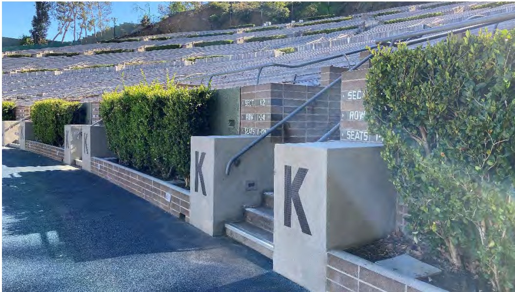
Photo 38 Typical horizontal aisle, or promenade, with section letter concrete buttresses and 1950s-era stacked concrete block planters in the seating area [48], looking east.
