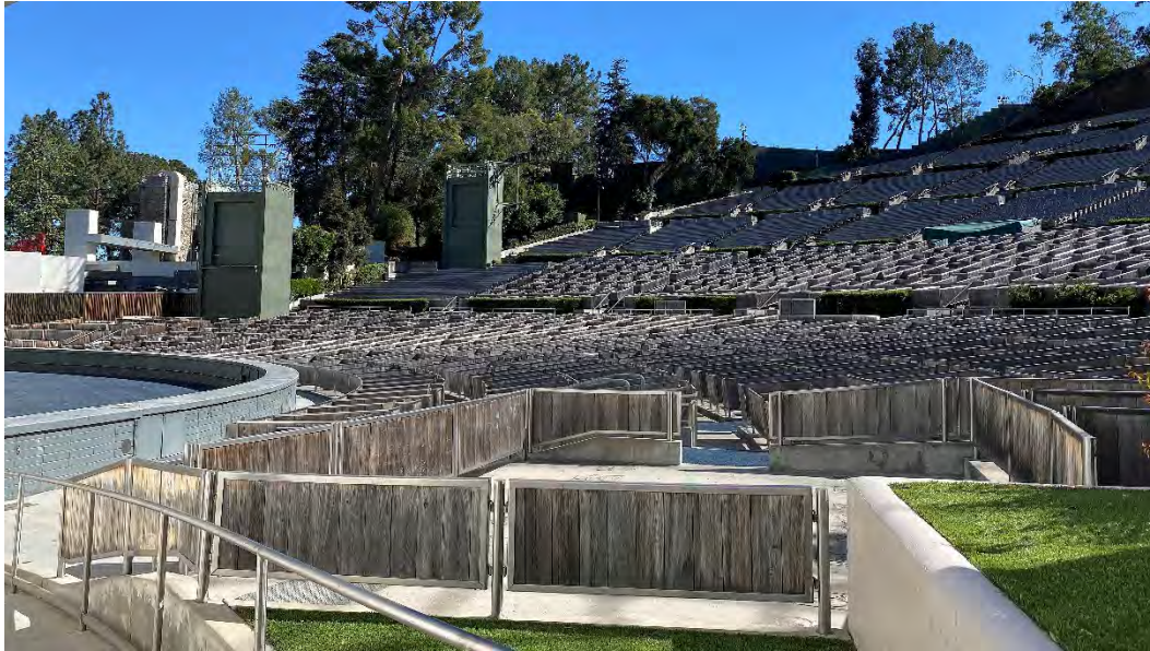
Photo 38 Typical horizontal aisle, or promenade, with section letter concrete buttresses and 1950s-era stacked concrete block planters in the seating area [48], looking east.
