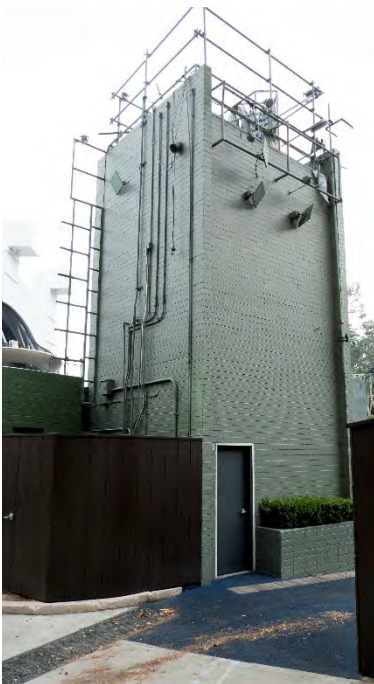
Photo 42 Detail view of rear and side of typical sound tower [49-52], with concrete blocks on the sides away from the stage.
