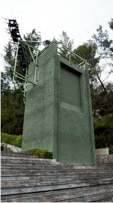
Photo 42 Detail view of rear and side of typical sound tower [49-52], with concrete blocks on the sides away from the stage.
